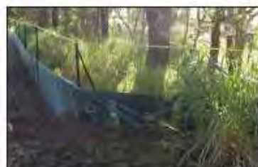
TREE PROTECTION & EROSION FENCE
